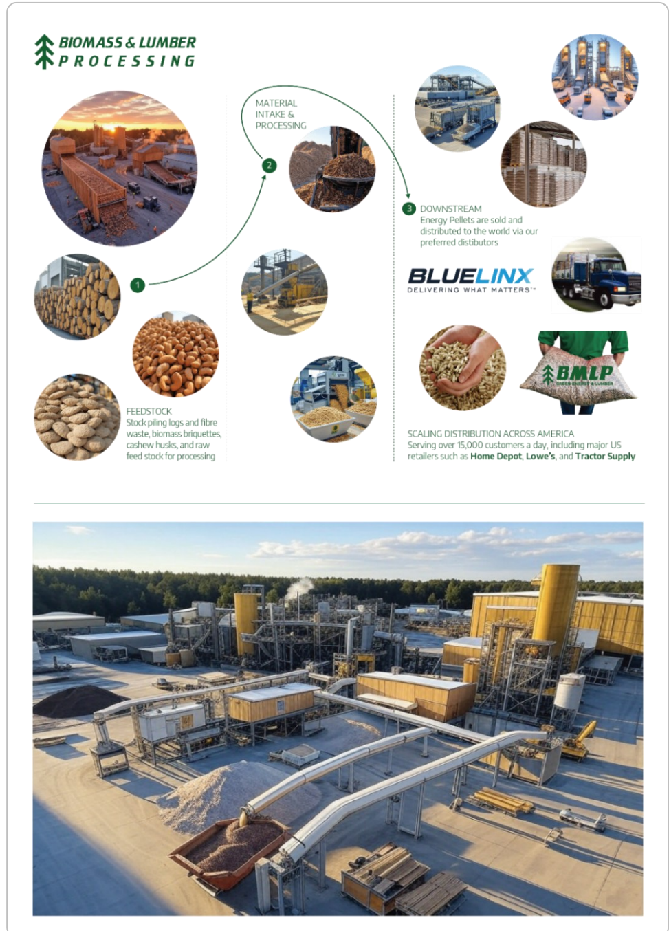
Figure 20: Closed-end loop system in practice: BMLP-BioMass facility
